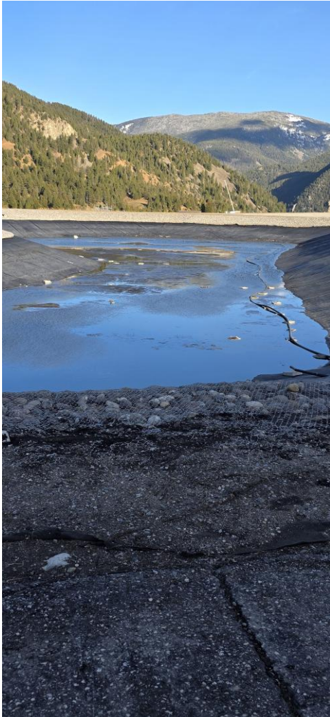
Aeration pond line removal
