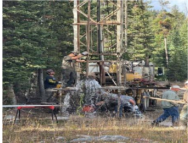
Sealing the casing of Test Well #9
