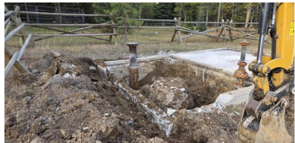
HV Well #2 Foundation Removal
