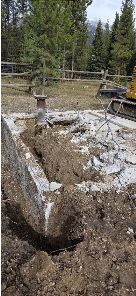
Hidden Village Well #2 Foundation Removal
