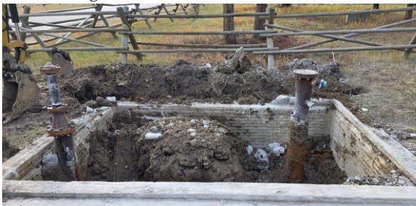
HV Well #2 Foundation Removal
